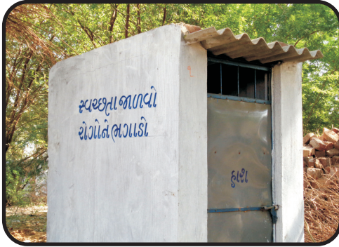
Toilet build at Jhagadia
